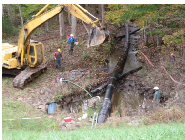
Above : “ Principal spillway slip line operations November 2021
