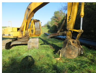
Above : “ Principal spillway slip line operations November 2021
