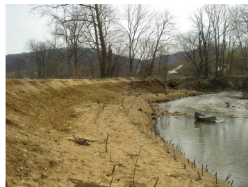
Left: Stream Bank sloped, bench and toe planted with live stakes Right: 5 years of growth, live stake willows
