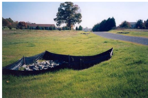
Example of stabilization with vegetation and outlet protection.
