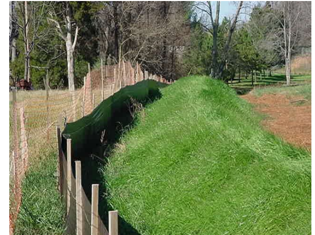
This is an example of diversion dike and silt fence. Note the vegetative stabilization on the dike.
