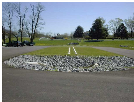
Stabilization with vegetation and outlet protection
