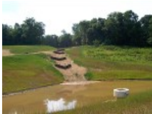
Figure 1: Active Erosion Control: Slope Remediation and Sediment Basin
