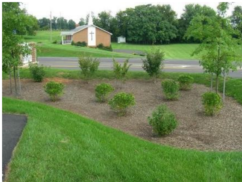
Figure 2: Bioretention Basin for the Farm Credit in Culpeper County
