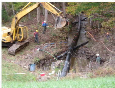
Above : “ Principal spillway slip line operations November 2021
