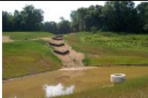
Figure 1: Active Erosion Control: Slope Remediation and Sediment Basin
