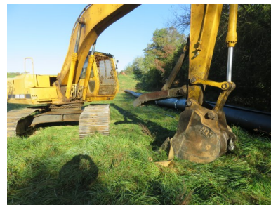
Above : “ Principal spillway slip line operations November 2021
