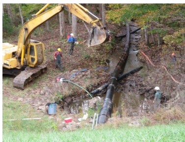
Above : “ Principal spillway slip line operations November 2021
