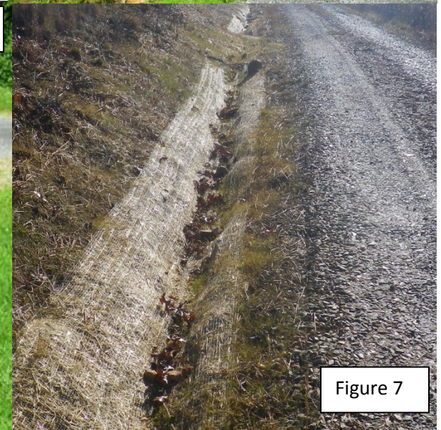
Figure 5: Elevated (In-slope) Gravel Driveway to inside ditch.
