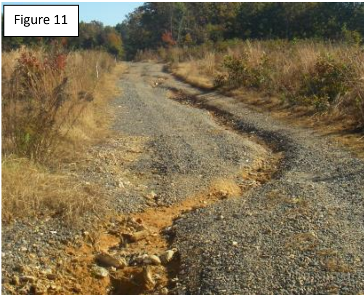
Figure 11: Lateral erosion across the roadbed, see #2.
