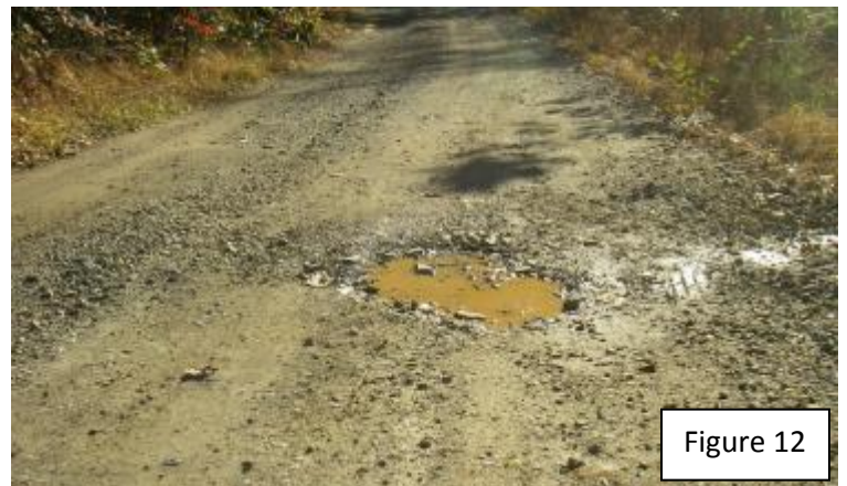
Figure 12: Common pothole in tire wear tracks. Formation can be due to poor soils or freeze/thaw action or shade prevents the area from drying out, see #5.
