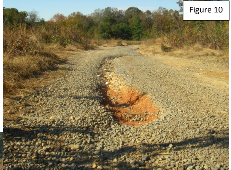
Figure 10: Erosion down the roadbed, see #1.
